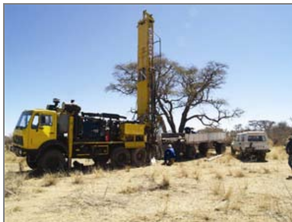
First drill hole, August 2007
