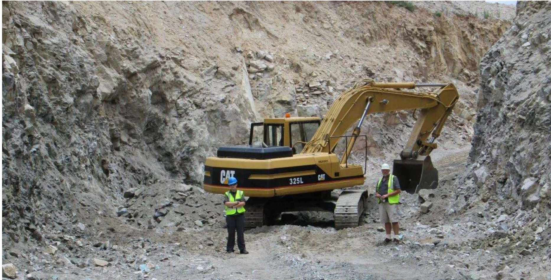
Excavating the oxide copper bulk sample pit, November 2012
