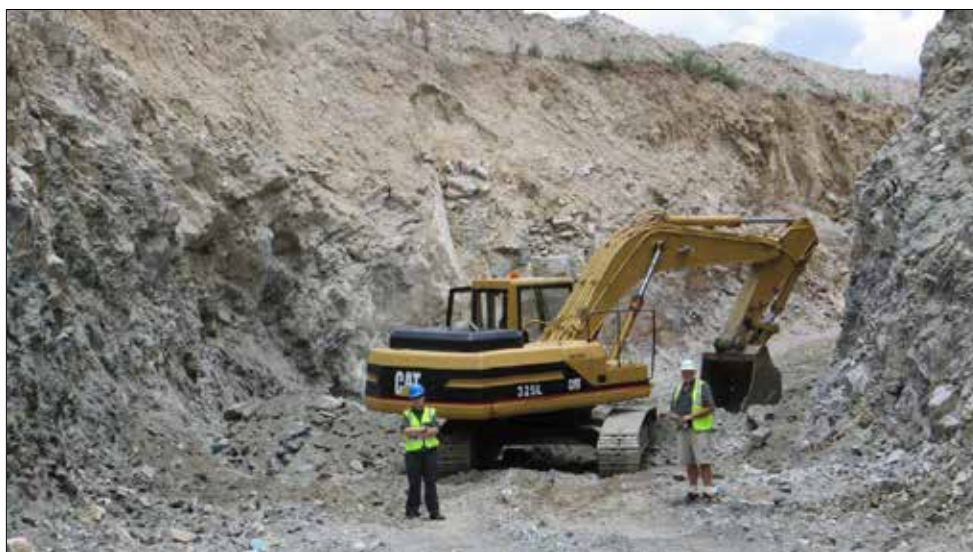
Photo 3. Excavating the bulk sample pit.
