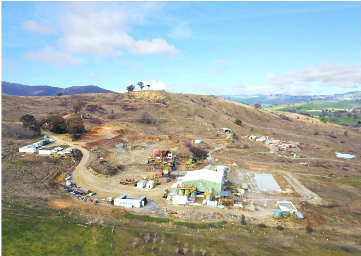
Aerial view of the Adelong Project site: Processing plant in the foreground, crushing circuit immediately left behind it. The portal to the adit is behind the buildings in the top right of the photo. The site office is at the back left of the photo.
