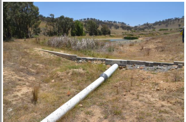
Plate 4 Goodwin Dam spillway outlet (Ref: E503B_063)
