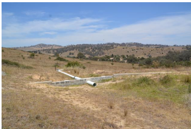
Plate 1 Goodwin Dam spillway (Ref: E503B_059)
