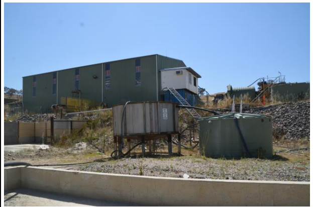
Plate 14 Processing shed (Ref: E503B_155)
