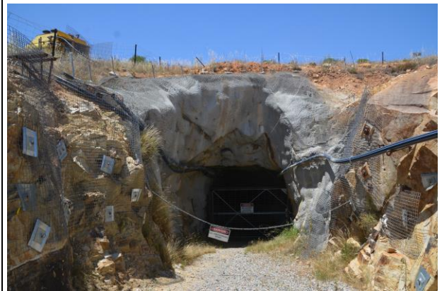
Plate 10 Decline portal into underground workings (Ref: E503B_068)
