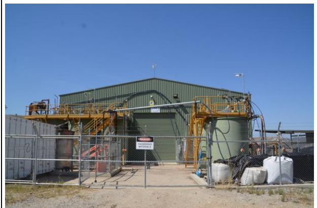
Plate 12 Processing shed (Ref: E503B_147)
