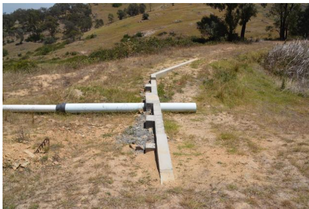
Plate 3 Goodwin Dam spillway outlet (Ref: E503B_061)
