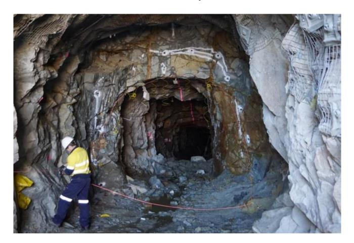
Step one measure and mark up, then drill the tunnel "face"
