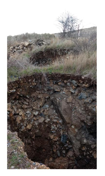
Rehabilitate vintage exploration holes left by previous companies. Filled with cement aggregate, preventing ground water issues.
